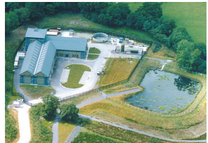
Example of remote pumping station.
