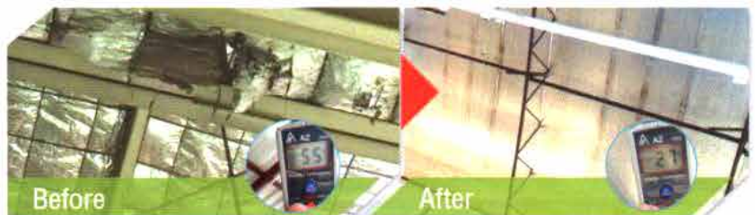
Replace the old Insulation
