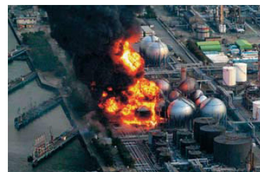
An explosion incident in hazardous area
