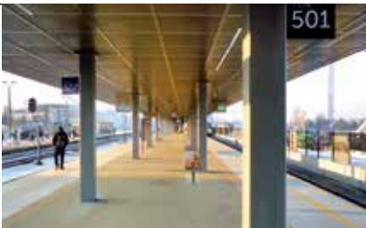
Railway stations Bahnhöfe
